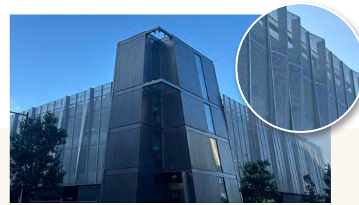
Sculptural aluminium screens providing wind protection.
