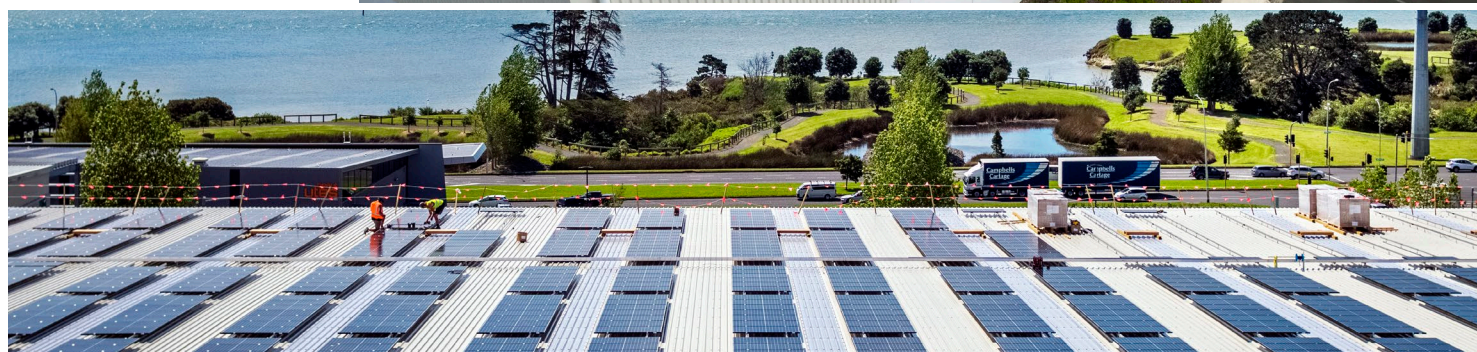
Installation of solar panels on the roof of the 7,500sqm warehouse extension(2021).
